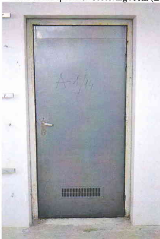
Photo No. 27655d-06
