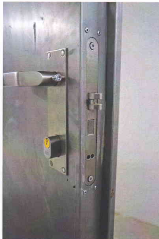
Photo No. 27655d-02
